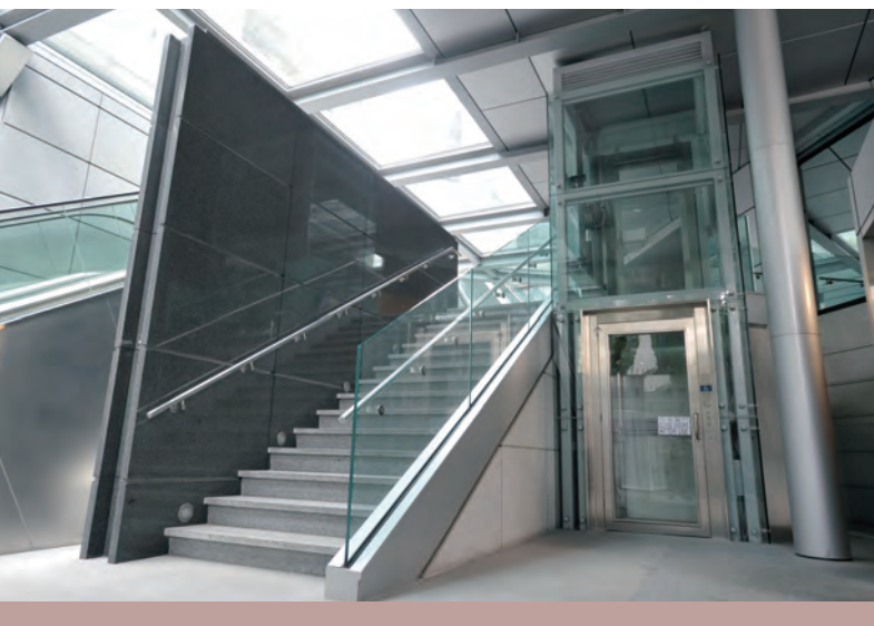
警察總部夏慤花園入口的無障礙升降機平台已經啟用。 The barrier-free lifting platform at Harcourt Garden entrance of Police Headquarters has been installed.
