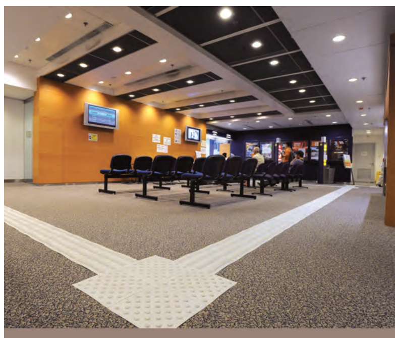
警察總部中央交通違例檢控組查詢櫃檯已加設觸覺引路徑。 A tactile guide path has been installed in the Central Traffic Prosecutions Division Enquiry Counter at Police Headquarters.
