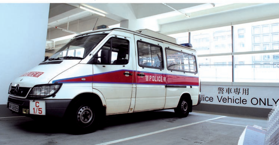
新中區警區總部大樓停車場的矮牆設計有助空氣流通。 The low perimeter wall design of the car park at the new Central District Headquarters facilitates better air ventilation.
