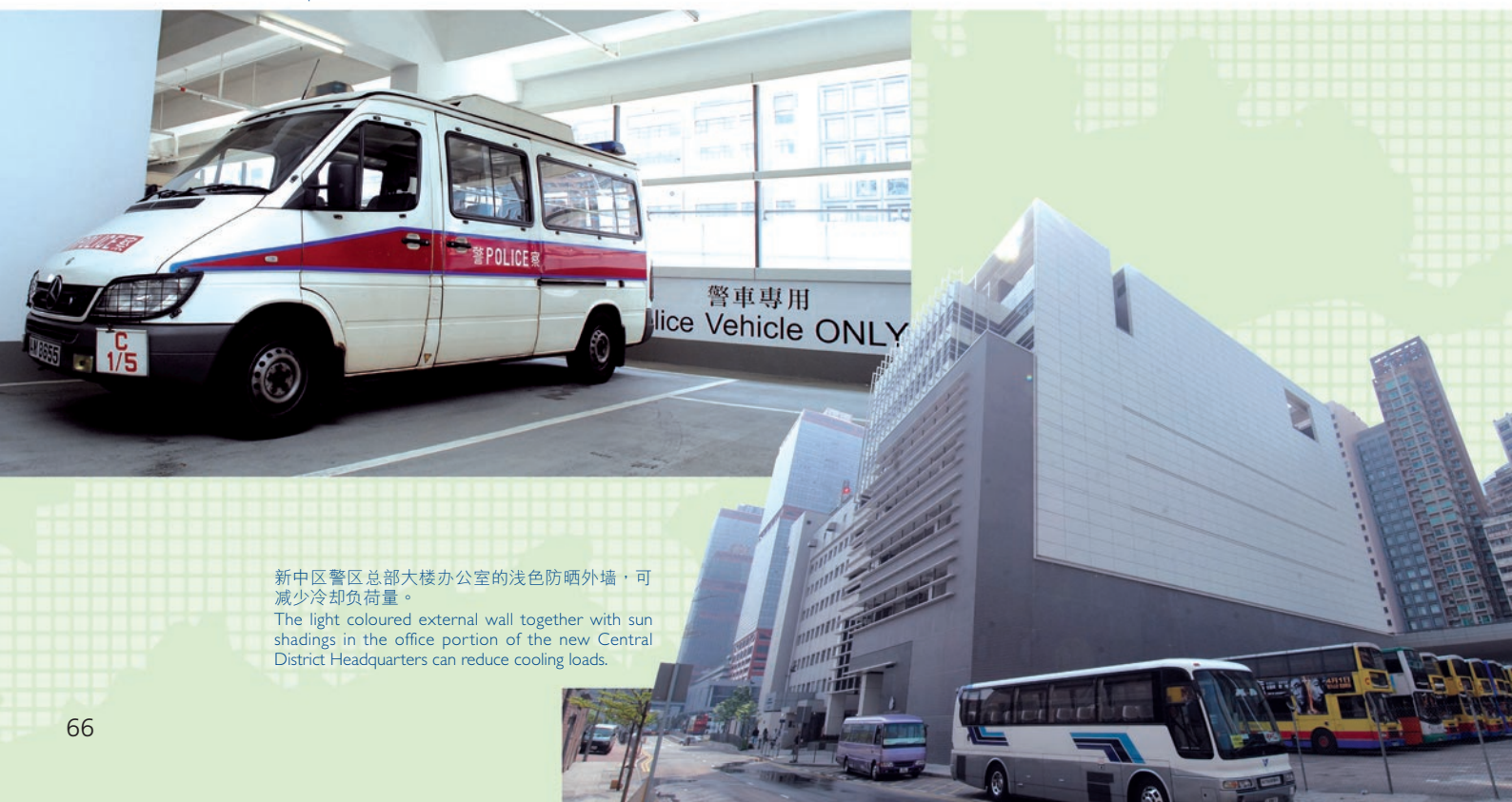
新中区警区总部大楼停车场的矮墙设计有助空气流通。 The low perimeter wall design of the car park at the new Central District Headquarters facilitates better air ventilation.
