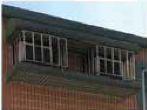
Air Conditioner Cage
