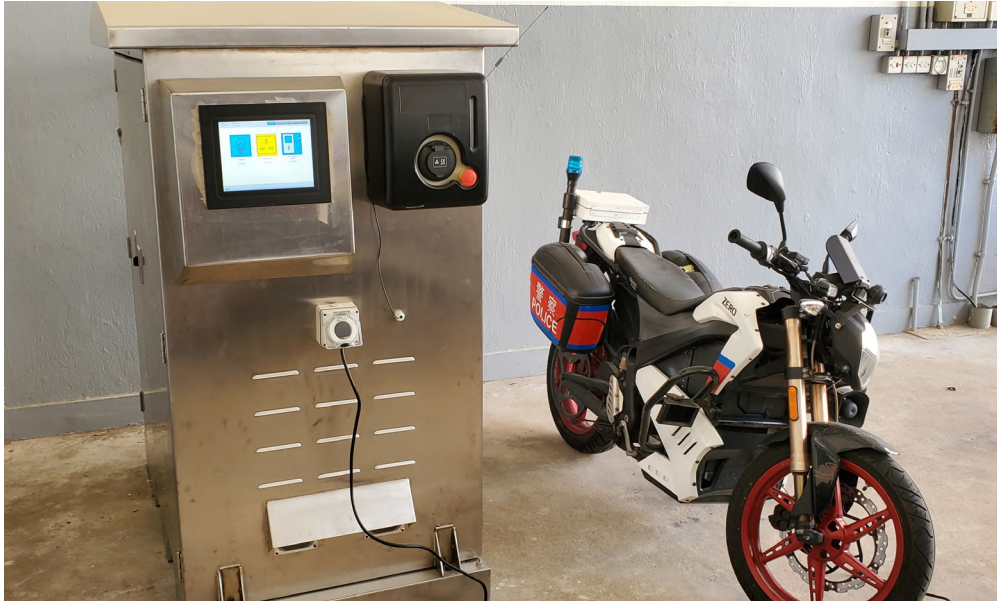
警察驾驶及交通训练中心设有电池储能电动车充电站。 The battery storage electric vehicle station in the Police Driving and Traffic Training Centre.
